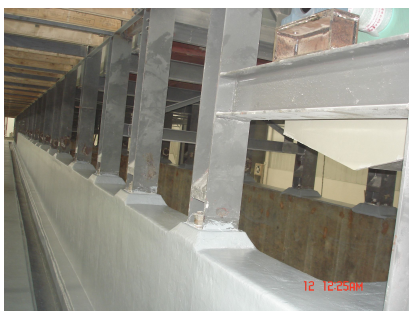
3. Protection of pickling tanks and trenches
