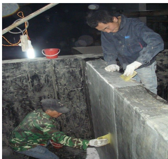
2. Lining of tank in fragrance workshop
