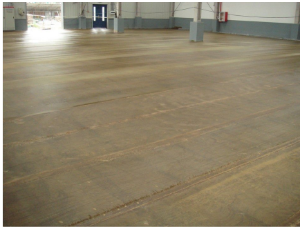
1. Floor for chemicals' warehouse
